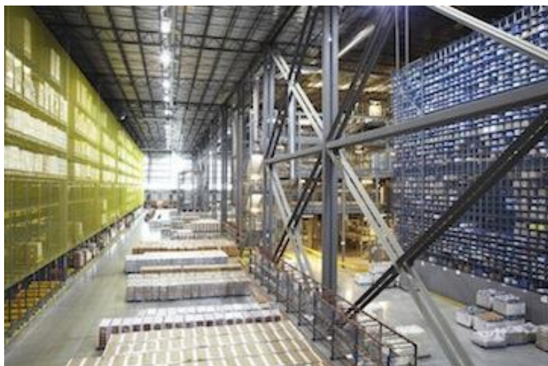
Figure 11 Sobeys Vaughan Automated Warehouse
